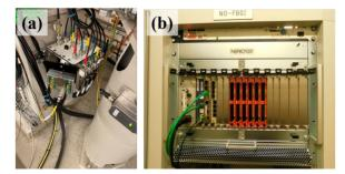
Figure 3: BPM readout system installation in PETRA III: (a) *Libera XBS FE* crossbar switch matrix installation in the tunnel and patch panel for signal splitting; (b) MTCA crate in the electronics cabinet equipped with 6 AMC boards, MCH, CPU, timing and fan module.
